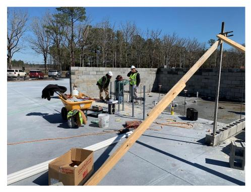
This picture of the group restroom in the eighth grade wing. This picture was taken on Wednesday. The boards are braces for the corner post the masons use to pull strings to lay the blocks to keeping the wall straight.
